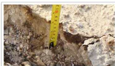
Figure 1. Crude Oil Penetration
