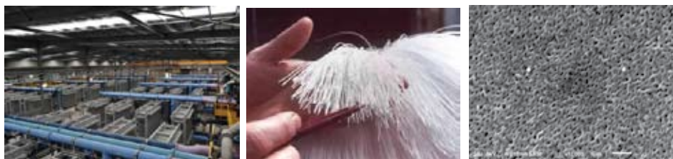
Figure 1. A 160 ML/day installation in Perth (left) uses MEMCOR's hollow fibre membrane technology (middle and right).
